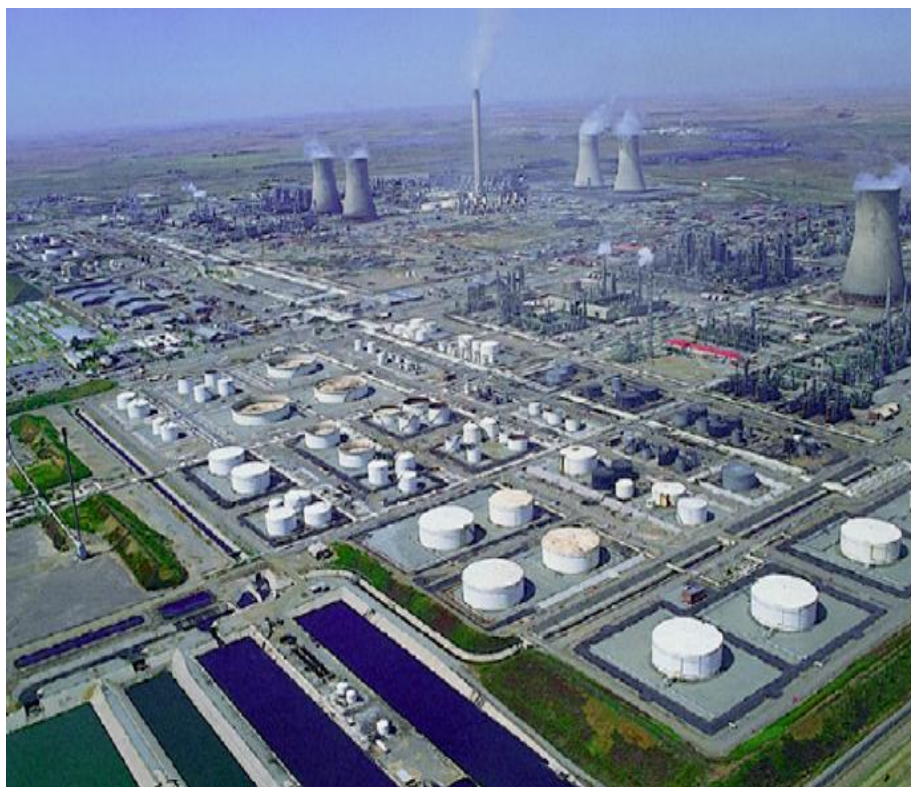
Sasol Coal-to-Liquids Plant Secunda South Africa
