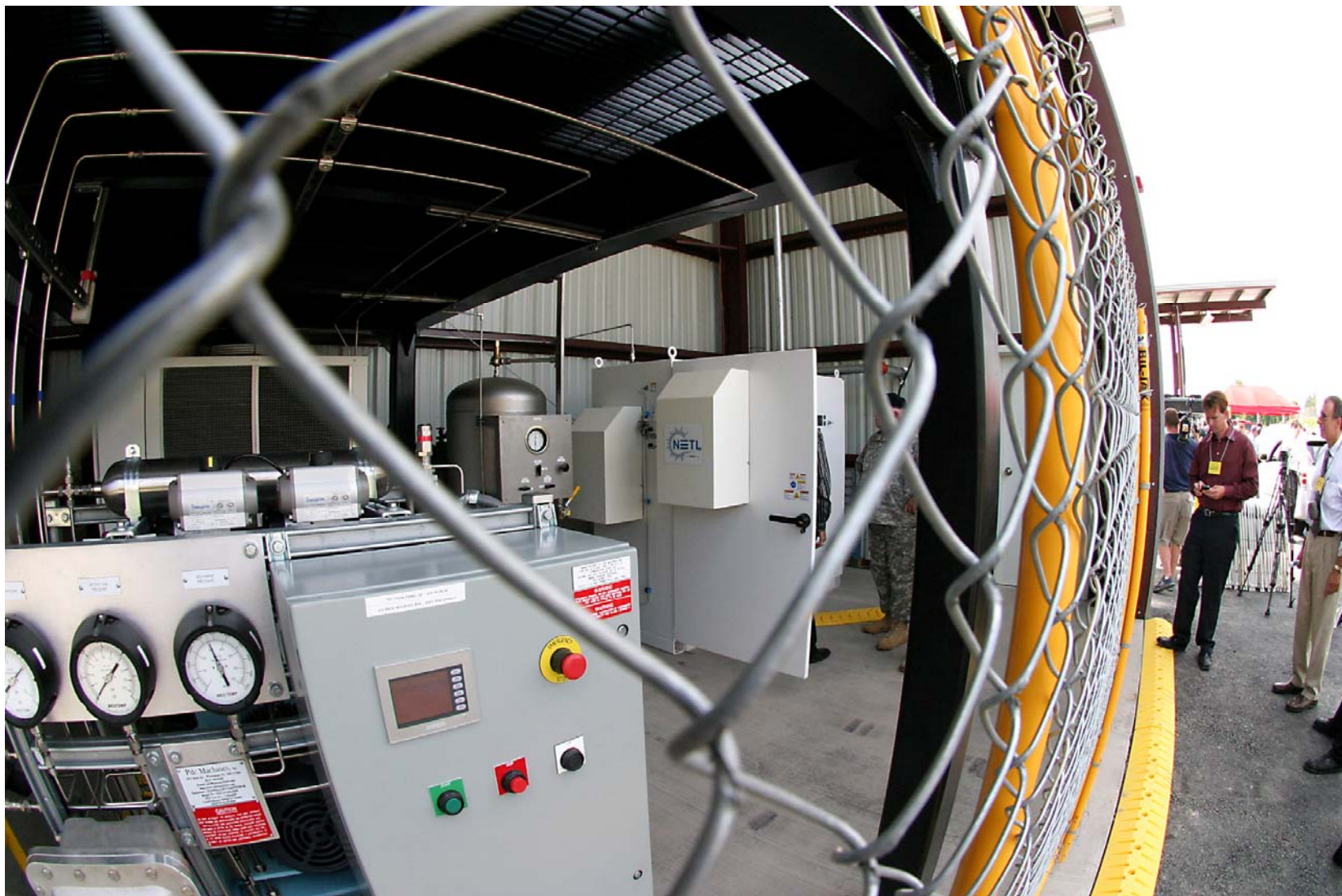
Hydrogen Production Uses Grid Power To Split Water
