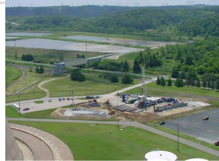
Drilling and Testing AEP#1 Well – 2003-05
