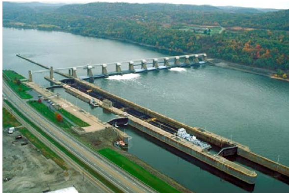
New Cumberland Locks and Dam
