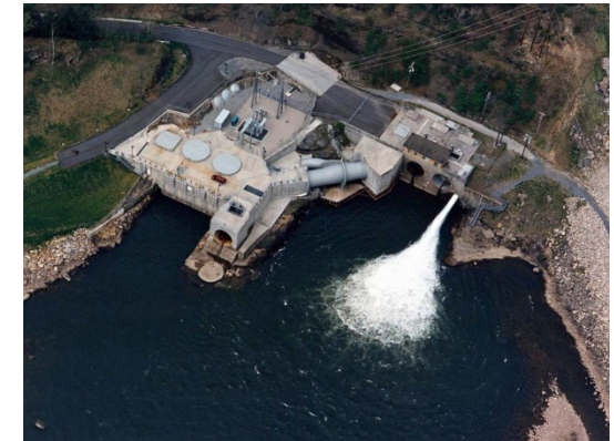
Hawks Nest Hydro Facility
